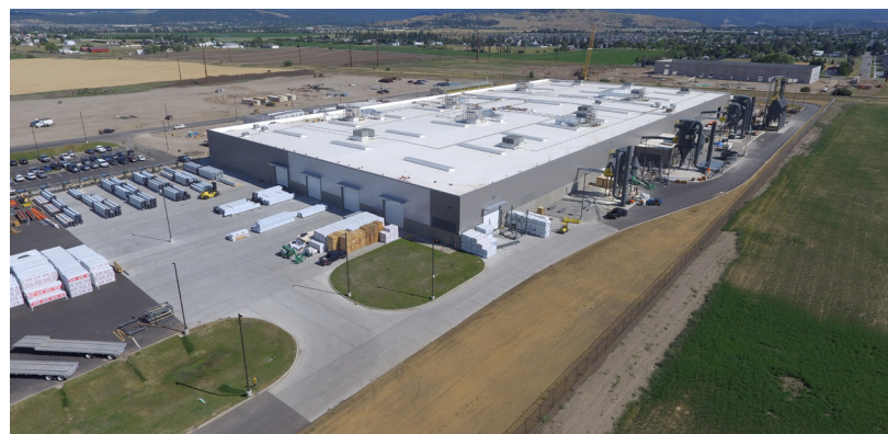
Katerra’s Spokane Valley, WA, CLT manufacturing facility is the largest in North America.
