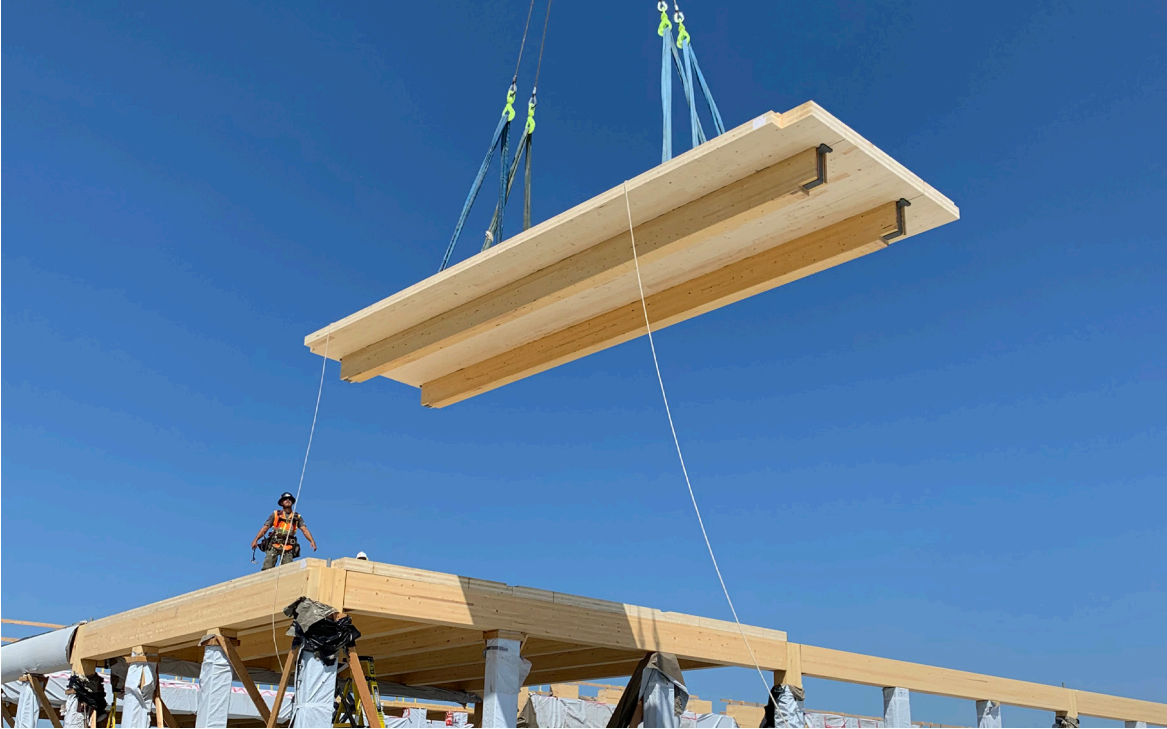
350 ribbed panels were prefabricated offsite and delivered to Catalyst.
