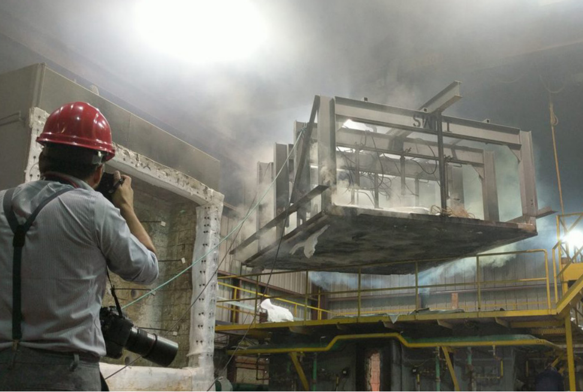
A load is applied for large scale horizontal furnace fire-resistive rating testing..
